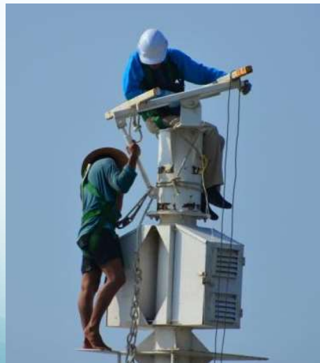
Tower No. 3 : Installation of solar panel
