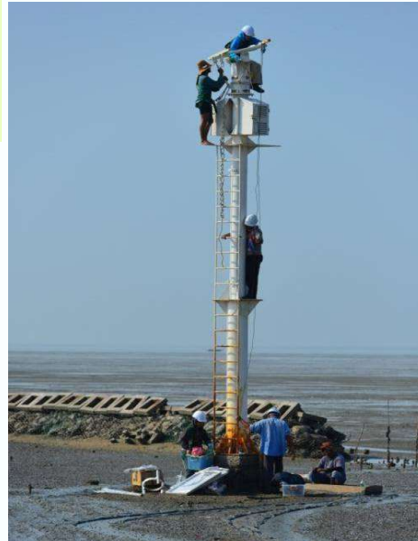
Installation of solar panel and control tracks
