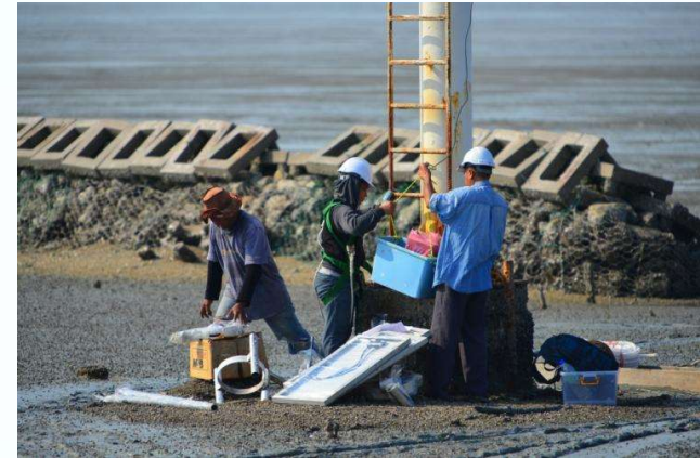
Installation of solar panel and control tracks
