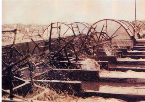
Mikawashima - Japan's oldest wastewater treatment plant in 1922
