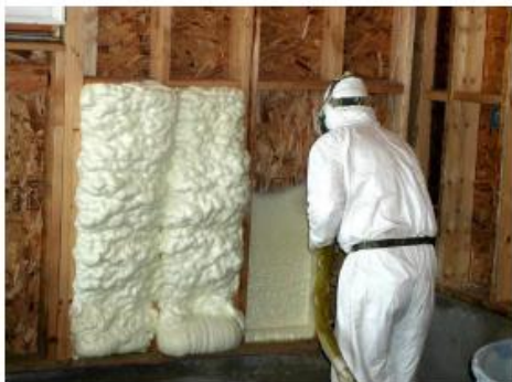
Spray foam installation
